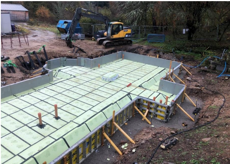
Construction of steel reinforcements for concrete foundations
