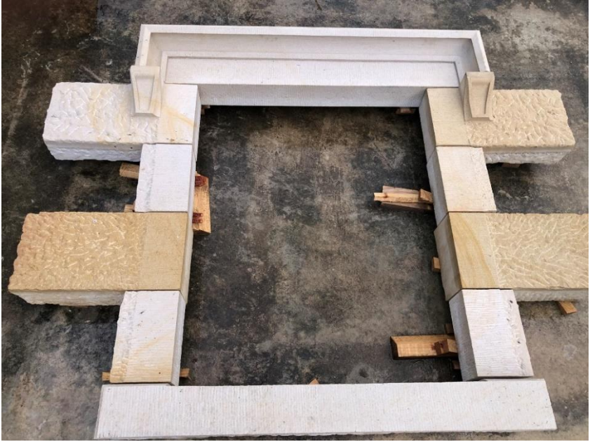
Complete window surround made by Andy Allan of Harper and Allan Stonemasons
