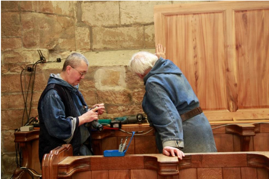
Br Daniel & Robin MacDonald-Johnston installing new choir screens
